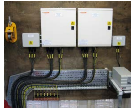
Power distribution, earthing and UPS for actuators and forklift charging point within a factory.
