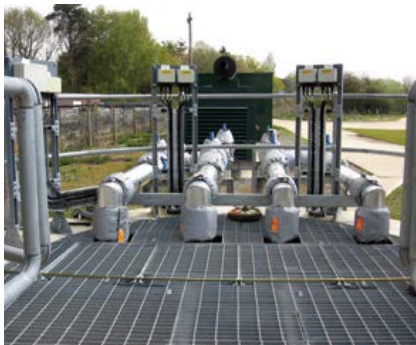
Power, control and instrumentation installed for a new wastewater pumping station and generator.
