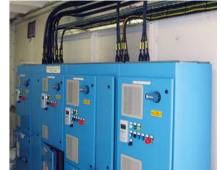
Installation of new MCC, cabling and containment work for a new wastewater pumping station.
