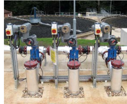
Cabling, containment and isolators for power and profibus driven actuators.
