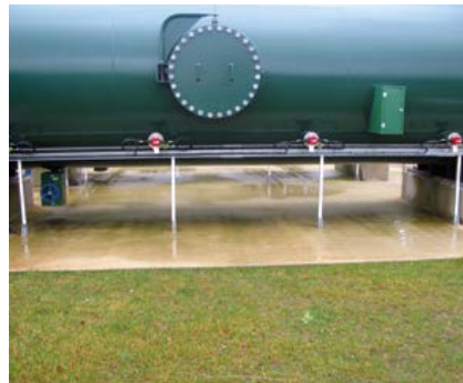
Cabling and containment for power supplies to heaters for a new surge vessel.
