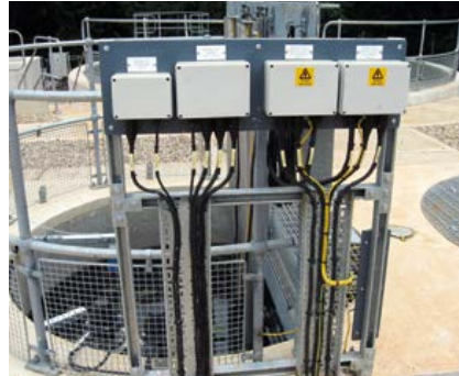
Cabling and containment for installation of instrumentation and motors for a new re-circulation pumping station.
