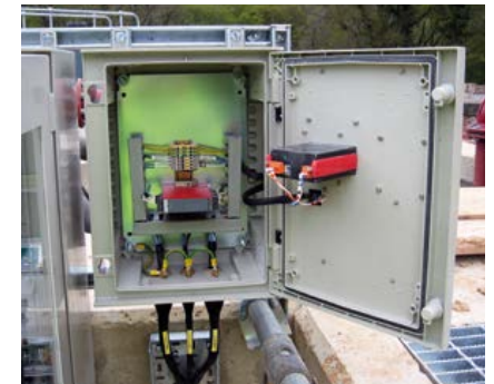
Cabling and cabinet for a Full Flow to Treatment MCERT flowmeter repeater for the EA.
