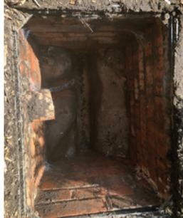
The specifications of the manhole used in this example are described in the table opposite. Based on this specification, should a downstream obstruction occur, the rate of rise will be fast.
