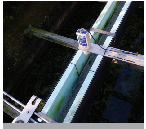
Final effluent location
